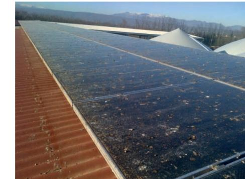
These pictures allow you to understand why the washing of the PV panels is so important. The dirt causes efficiency losses, while the big persistent spots can cause serious damages to the entire PV equipment.
